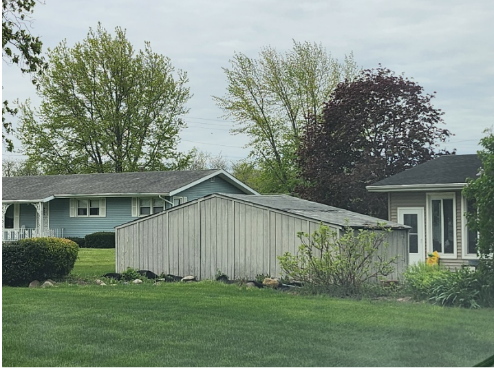
View from Bridge St
